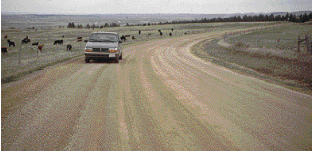
This superelevated road section makes driving safer.
