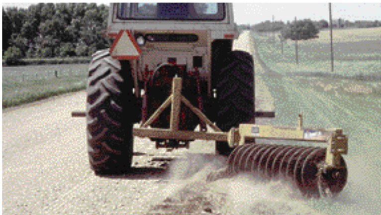
Same machine mounted on a farm tractor to help break up material on shoulder.
